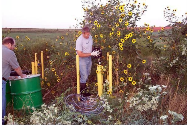
Figure 11 – Typical Monitoring Well Nest for Monitoring above and below the Production Zone
