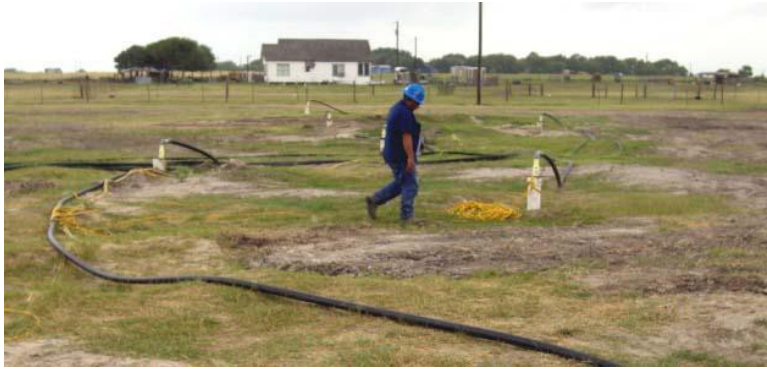
Figure 10 - Well Spacing of Injection and Recovery Operations at a Present Texas Operation.
