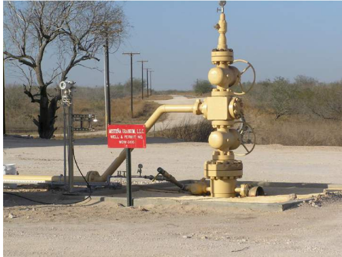
Figure 29 – One of MULLC’s Waste Injection Wells.
